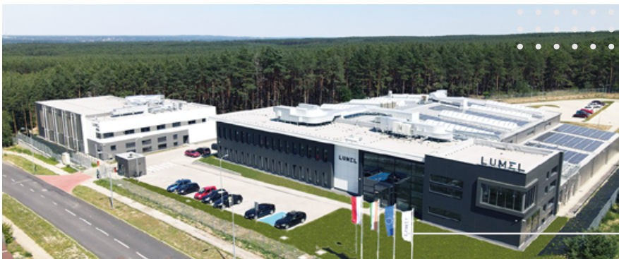
Plant area 3.650 m 2 powered by Lumel solar installation
